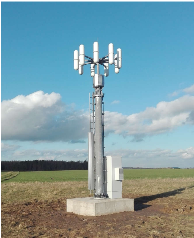
Field installation of the IZT R5509 direction finder in Calden.
