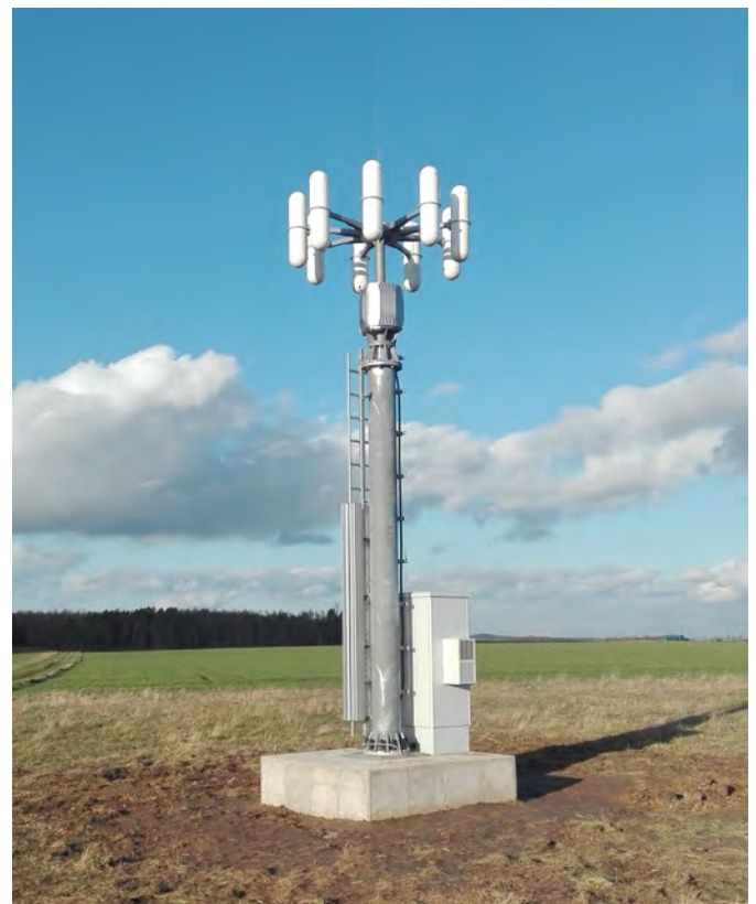
FIGURE 2: CUSTOMER INSTALLATION WITH IZT DF ANTENNA AND RECEIVER
