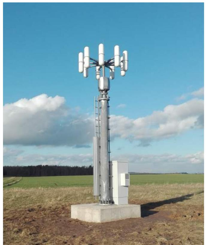
**FIGURE 2:** CUSTOMER INSTALLATION WITH IZT DF ANTENNA AND RECEIVER
